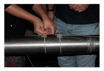
Figure 1.3: Installation of ultrasonic flowmeter transducers/receivers
