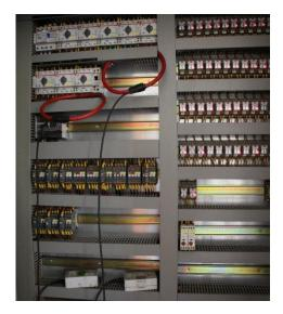
Figure 1.7: Two current clamps installed in an electric board
