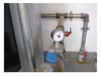
Figure 1.5: Pressure gauge in a domestic hot water system
