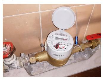
Figure 1.1: Nutating disk flowmeter
